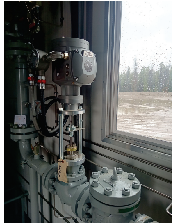
Bear BAL-6L Linear Actuator mounted on a ET style back pressure valve
